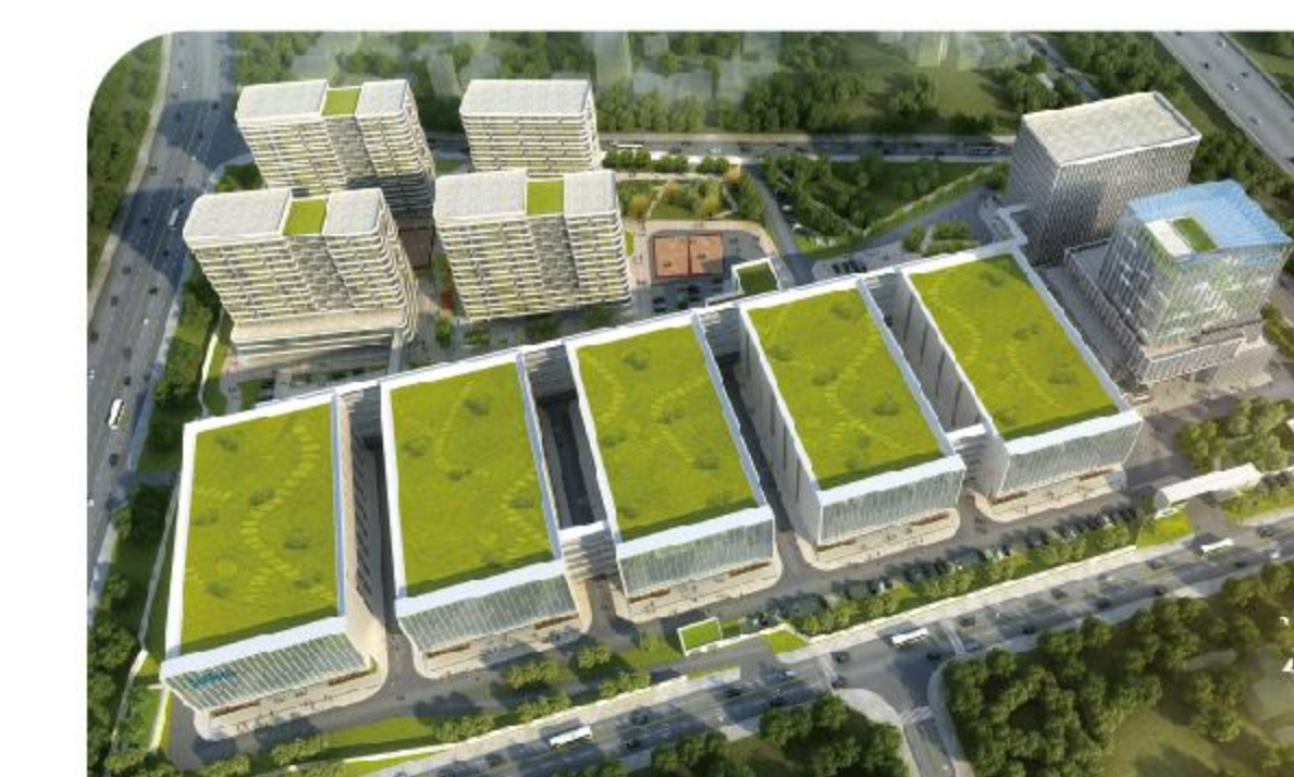
● 顺络新型电子元件及精密陶瓷项目基地 (东莞塘厦建设中) Sunlord New Electronic Components and Precision Ceramics Project Base (under construction in Tangxia, Dongguan)
